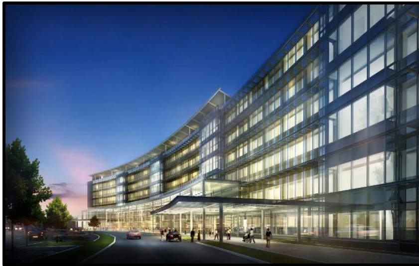
Figure 2: Evening view of south facade looking west
